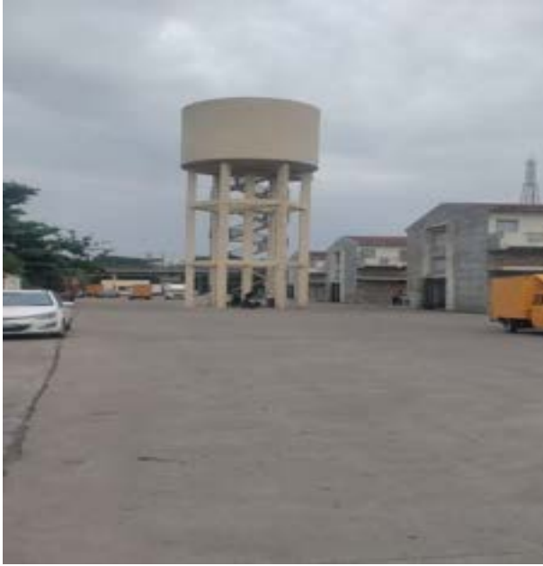
Overhead Water Supply Tank
