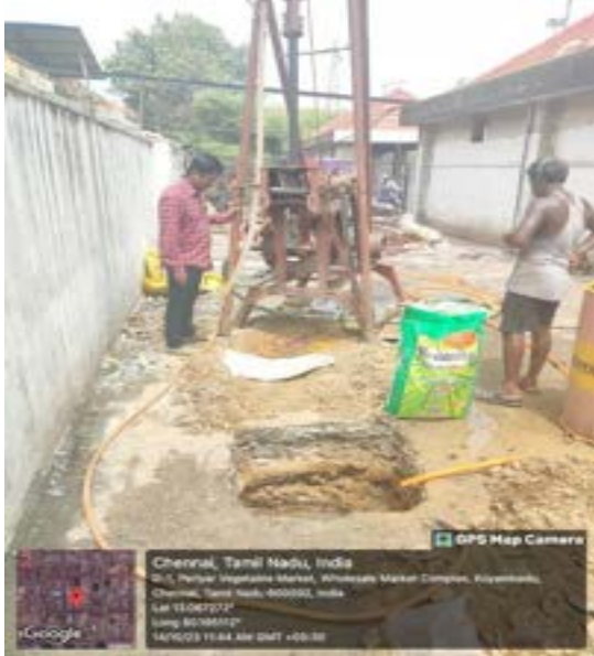
Fig. 7.10: Borewell preparation work
