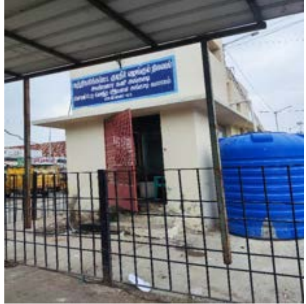
RO Plant pumping station
