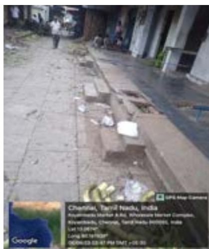
Fig. 7.2: Exterior of drain connection
