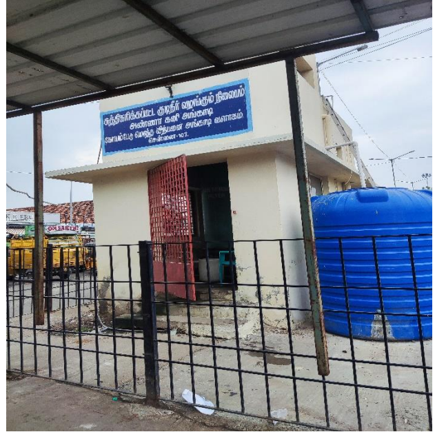
RO Plant pumping station
