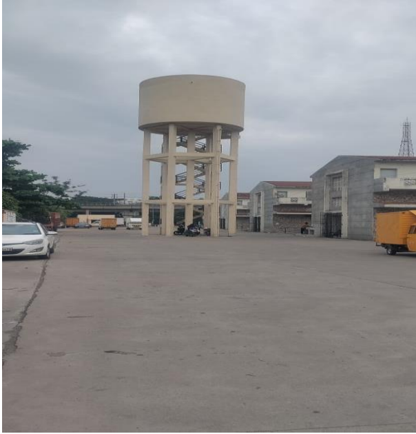
Overhead Water Supply Tank
