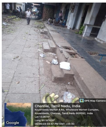
Fig. 7.2: Exterior of drain connection
