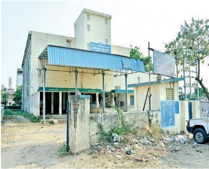
Cold storage complex
