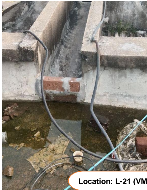
Fig. 8.6: Deterioration of the roof structure
